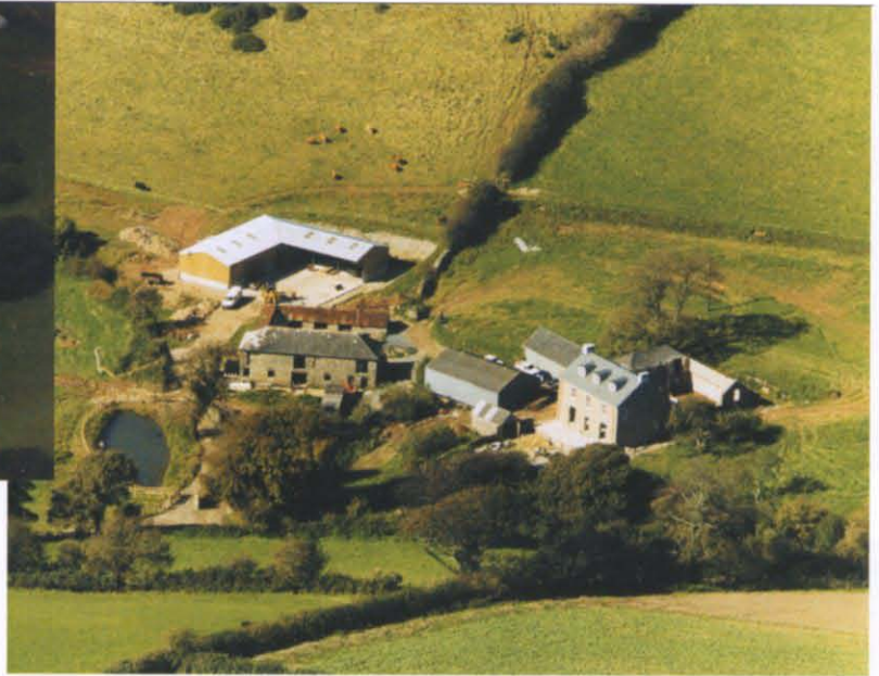
7. Aerial view before work began
